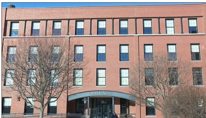
Developers look to transform a vacant mill in downtown Lewiston, ME, into an AI data center.
