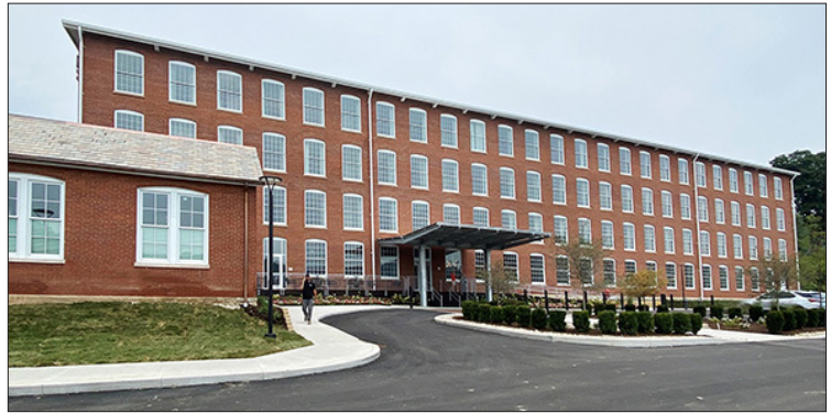
Eagle Cotton Mill Fairfield Inn & Suites received Indiana Landmarks’ Renaissance Award, which recognizes the revitalization of “long-decaying historic properties.”
