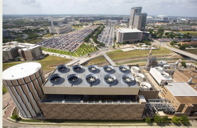
Figure 5.11. The Thermal Energy Corporation (TECO) district energy system (Texas Medical Center)
