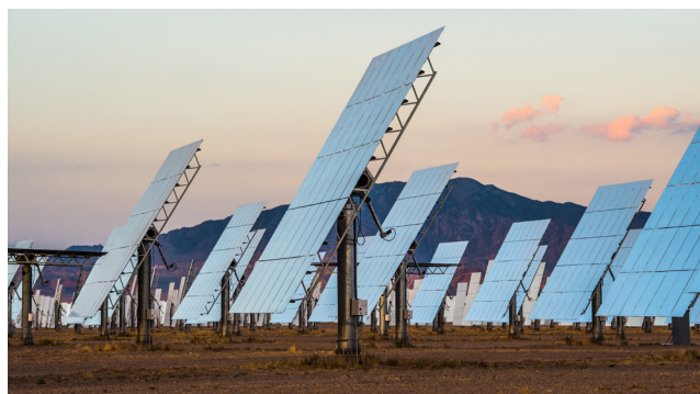
Figure 6.1. The Crescent Dunes Solar Thermal Facility in Tonopah, Nevada, uses solar photovoltaics and molten salt technology to provide renewable energy day and night (NREL/Flickr (CC BY-NC-ND 2.0))
