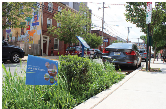
Figure 5.12. Green stormwater infrastructure installed as part of Philadelphia’s Green City Clean Waters, Green Street Program (Philadelphia Water Department)
