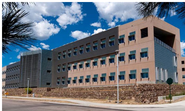
Figure 5.13. The National Renewable Energy Lab's research facility building features a transpired solar collector, or dark colored metal sheeting on the south side of the building that collects heat from the sun, on the building exterior as well as solar shading over the windows (NREL)
