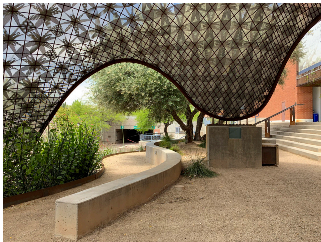
Figure 5.5. A shade structure designed and built by architecture students at the University of Arizona uses ventilation for increased air flow to help keep students and faculty cool (University of Arizona, CAPLA)
