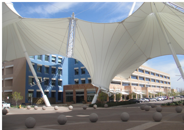
Figure 5.4. The Skysong Center in Scottsdale, Arizona, features dramatic shade structures, drought- and heat-tolerant vegetation, and building orientation for heat mitigation (Cygnusloop99/Wikimedia Commons (CC BY-SA 3.0))
