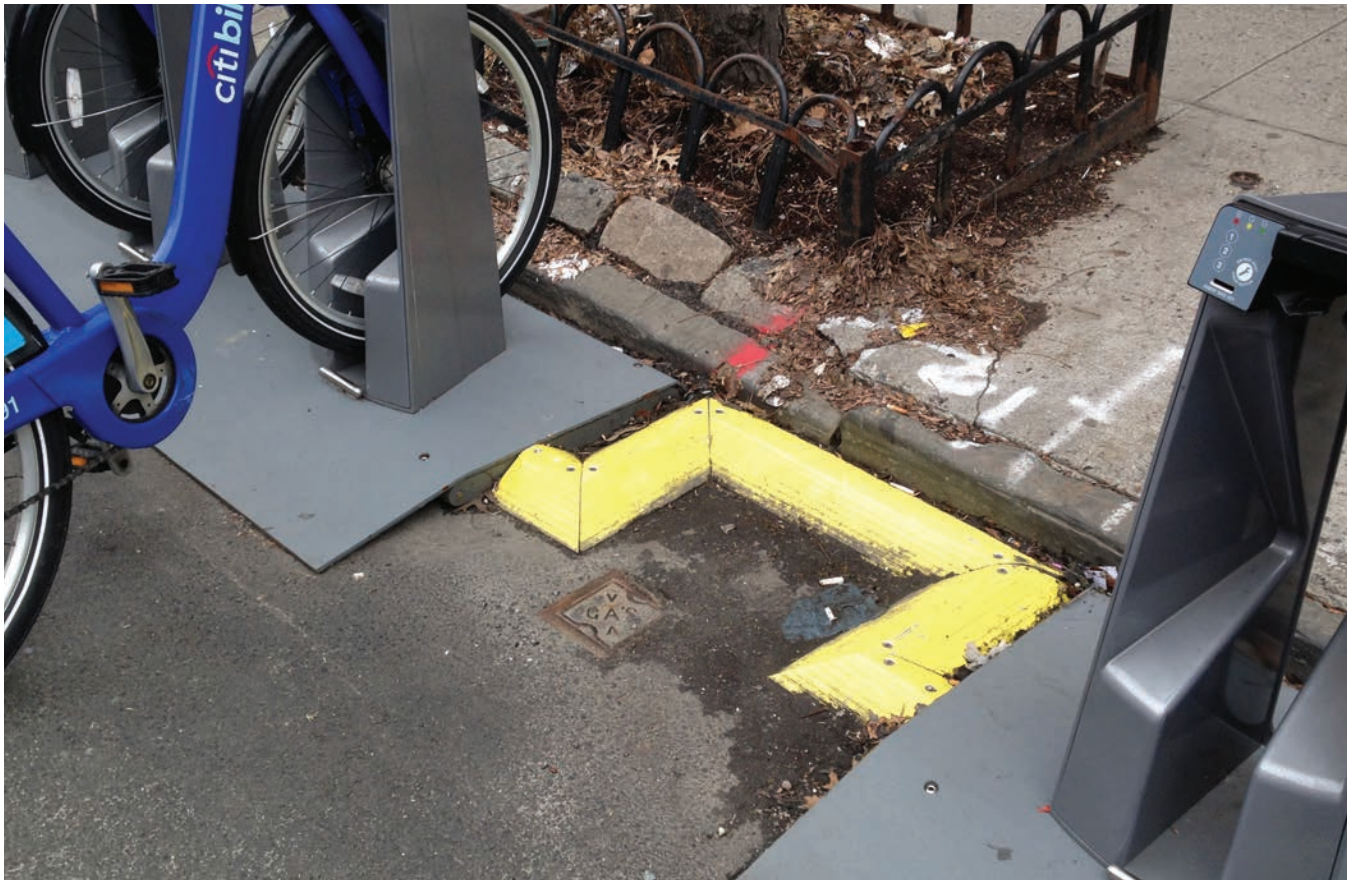
Bridging allows the station to fit around a utility cover and provides additional flexibility in station design. Citi Bike. New York, NY Photo: Kate Fillin-Yeh/NACTO
